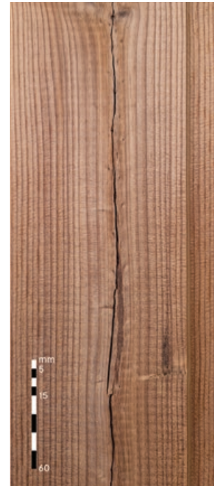
Surface cracks A grade: Allowed, up to 150 mm long B grade: Allowed, unlimited
